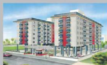
Residencial Ville de France CCSW 4 - Lote 2 - Setor Sudoeste Brasília-DF
